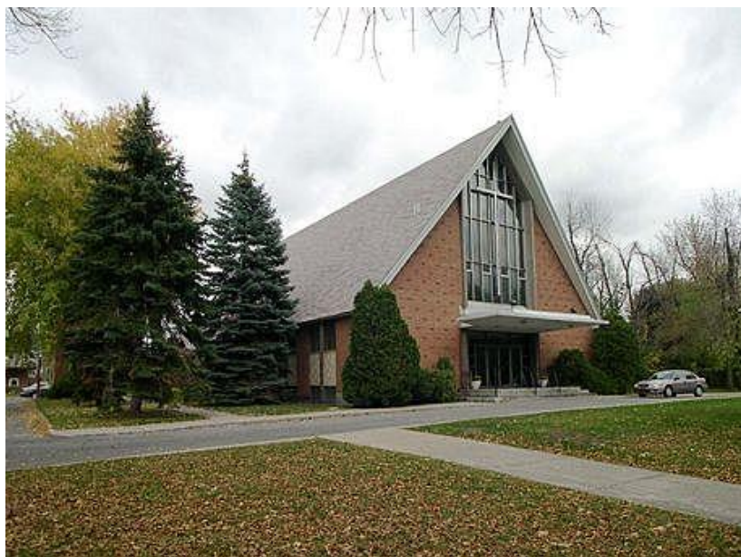
St. Francis of Assisi's Church
